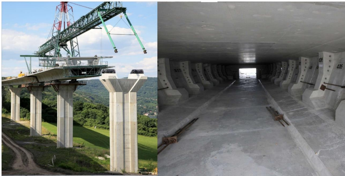
Fig. 1. Segmental construction approach applied at the D8 highway project in 2014. (Source: ŘSD ČR (Directorate of the roads and highways of the Czech Republic))
