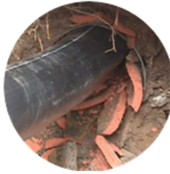
Figure 3 (b). Pipe bursting operation. (A-1 Trenchless Services LLC, 2017)
