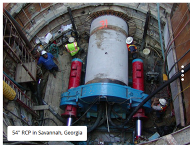
Figure 2. Microtunneling launching pit with Equipment setup. (BRH-Garver Construction, L.P., 2017)
