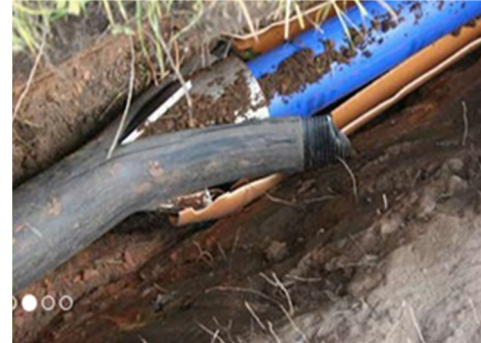
Figure 3 (c). Pipe splitting operation. (A-1 Trenchless Services LLC, 2017)
