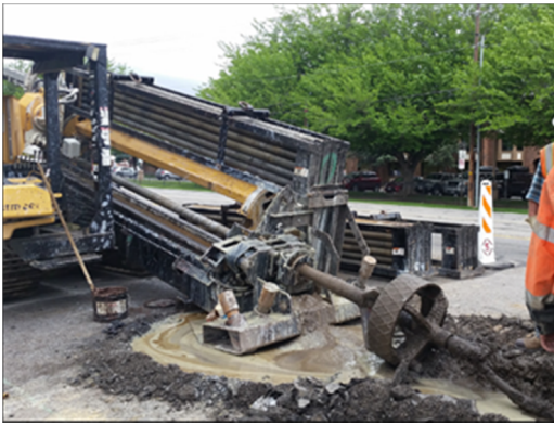
Figure 1. (a) HDD Rig setup. (Intermountain Drilling Supply, 2017)
